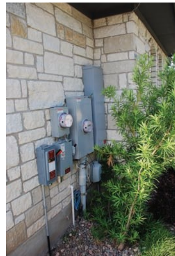
FIGURE OCCUPATIONS 6 One meter records the power supplied by the utility company, and another records the amount of power supplied by the solar panels.
